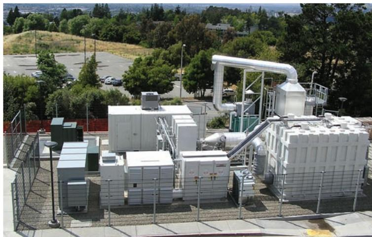
Fuel cell with heat recovery used for hot water heating at a university.
