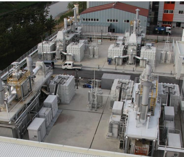
A 11.2 MW fuel cell installation in South Korea with thermal energy sold to a neighboring wastewater treatment facility
